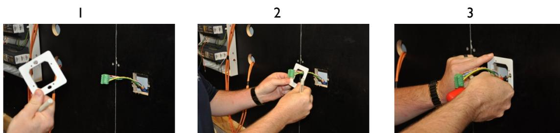
4. Ensure that the mounting plate is level and adjust if required.
