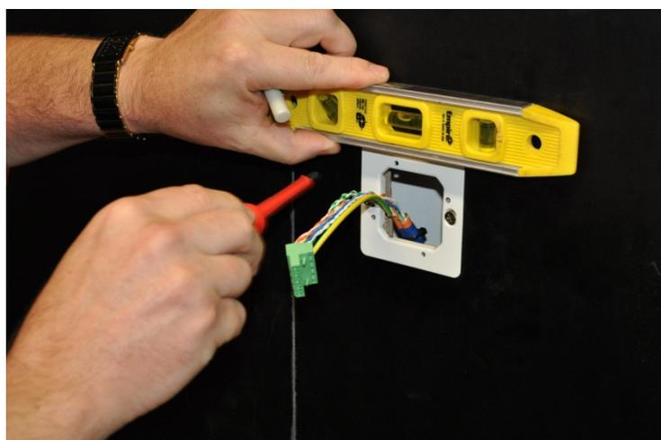
5. Once the mounting plate is secured, plug the phoenix connector into the communication module. If the communication module is not already attached to the application module, attach it now.
