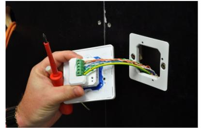
6. Push the panel assembly into the mounting bracket. Locate and fix the application unit to the mounting bracket using the two smaller screws through the mounting holes. Recheck the level of the panel and adjust if required
